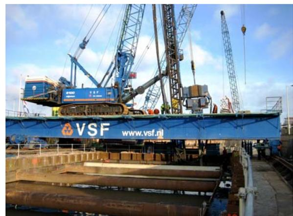
**Figure 1: Piling rig**
