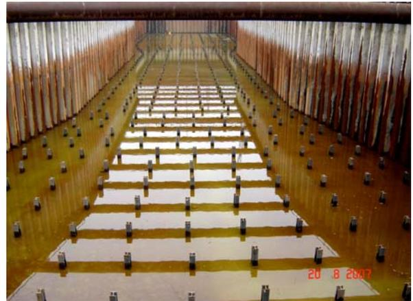
**Figure 11: The building after almost complete dewatering**
