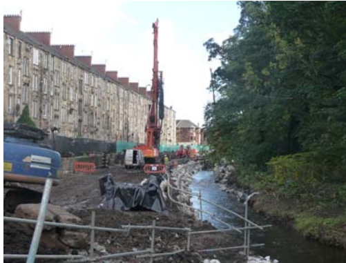
Figure 8. Execution of piling works.
