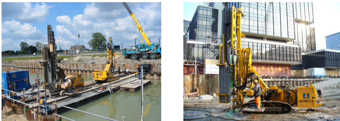
Figure 4. Pile installation.
