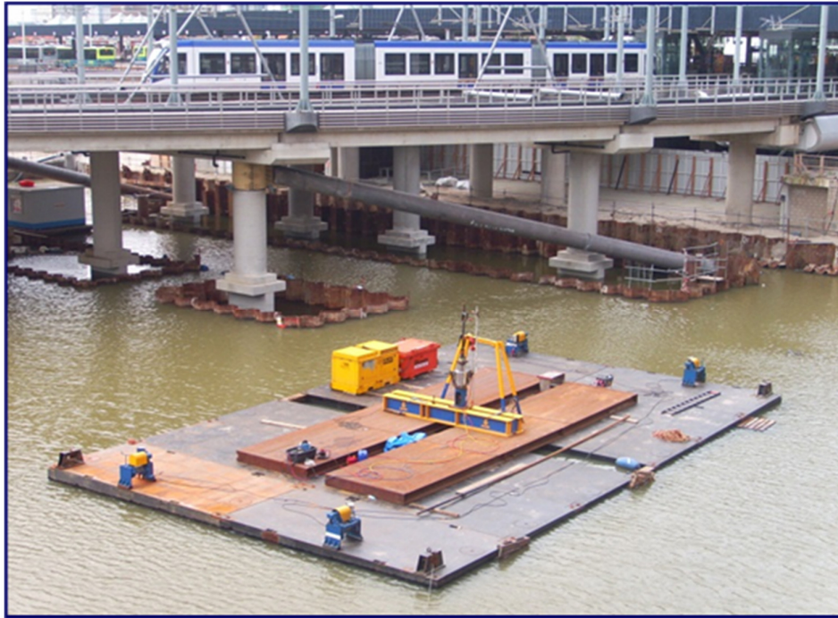
Figure 14. Suitability test conducted from pontoon after wet excavation of the construction pit.
