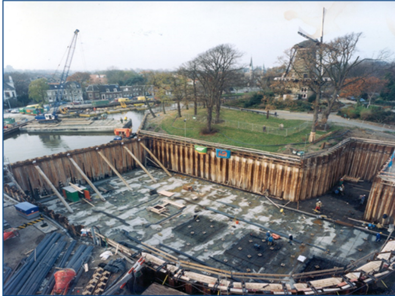
Figure 1. Construction of underground car park in the city of Alkmaar.
