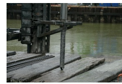
E Vibrated with temporary steel casing
